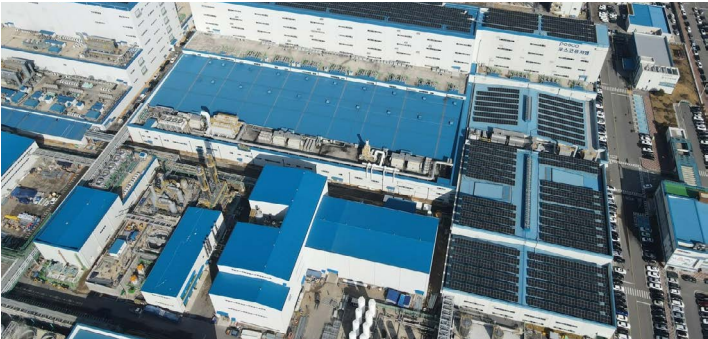
Gwangyang Cathode Materials Plant solar power facility
